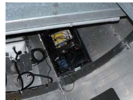
Remote microphone installed at the nacelle's bottom (above) and connected to automated bat detector inside the nacelle (below). © L. Bach
